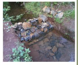
width. This method is effective where the depth of the stream is not more than one and a half meter and the sides of the stream are of clay. On the upstream side of masonry check dam at two to three places if these kinds of gully plugs are constructed then they prevent land erosion. Moreover they check sediments from entering into the dams and increase the lifespan of downstream structures
